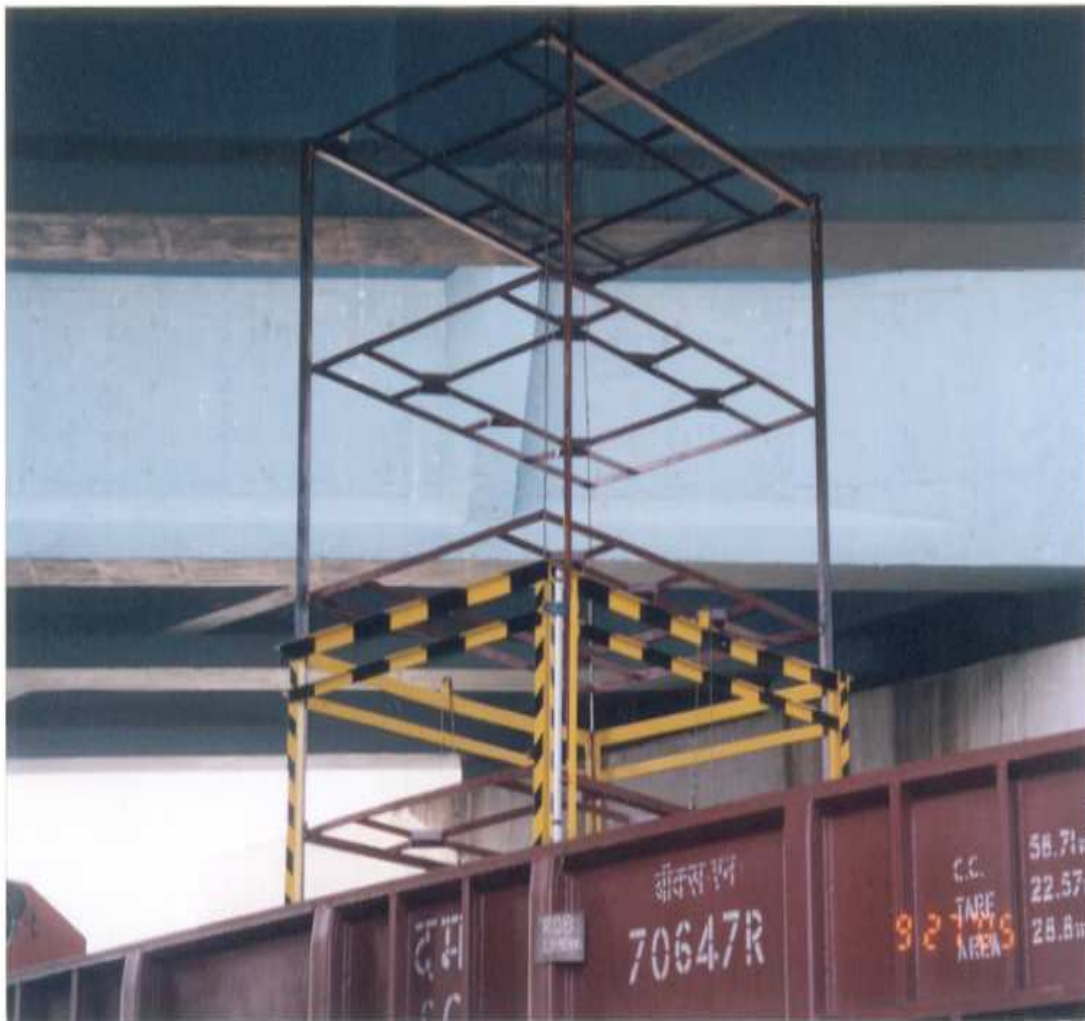
PHOTO of BOX Structure
